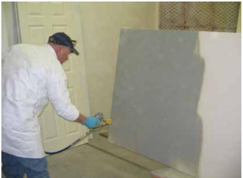
dried to a uniform olive green colour, approximately 45 to 90 minutes at 21°C, visually inspect the coating for any voids or pinholes. Fill any defects with additional material and apply the second coat at right angles to the first. The wet film thickness should be checked periodically using a wet film gauge. Each wet coat should be 0.4 – 0.6 thick. The combined dried coating should be 0.5 - 0.8 mm thick.
